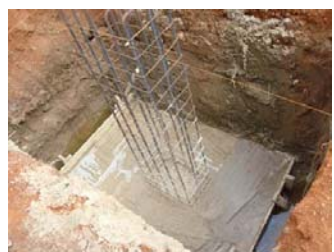
Proper Footer & Rebar
