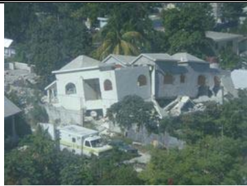
Still Many Damaged Homes..
